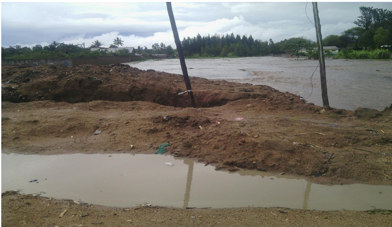
Figure 7: Showing seasonal river reclamation at Musoma bus river bridge along Nyerere Road, Nyakato/Nyasho boarder. Source: Field Work, November, 2015.
